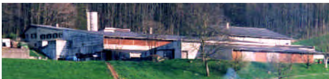
Links: Schweinefabrik in Gretzenbach
