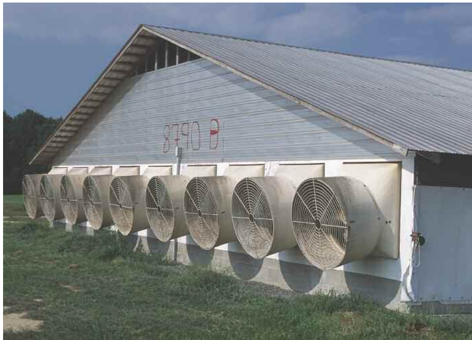
Adding more to the carbon footprint: large fans keep pigs cool in North Carolina.
